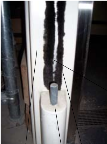
Door Frame Pivot & Guard Brush Seal
