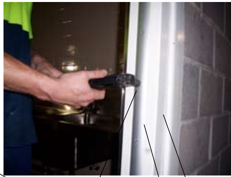
Pop Revit Seal To Door Frame Dome Seal Door Frame
