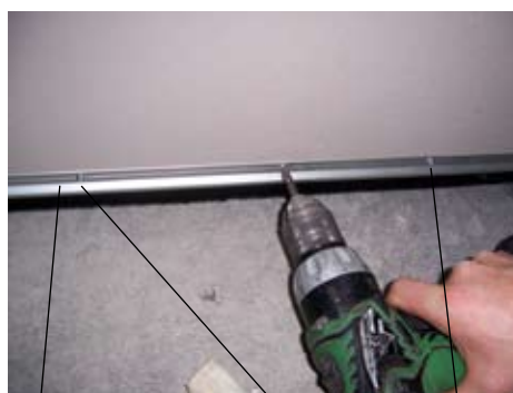
Brush Seals Attach Brush Seals With Screws
